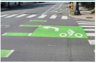
A **two-stage left-turn** box designates an area at a signalized intersection where bicyclists can queue in a right-side bicycle facility to increase comfort when making a left turn. Twostage left-turn boxes are typically provided when a protected or dedicated intersection is not feasible and the roadway experiences high vehicle volumes or a large number of bicyclists that make left turns.
