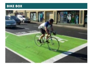
A **bike box** designates an area in front of the vehicular lanes at a signalized intersection. The bike box increases bicyclist visibility by allowing bicyclists to get ahead of queued vehicles during a red signal phase. This treatment can help avoid a "right-hook" conflict between bicyclists and right-turning vehicles.
